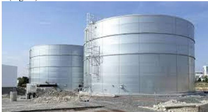
Fig. 1. Storage tanks for liquid substances.
