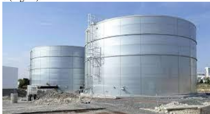
Fig. 1. Storage tanks for liquid substances.
