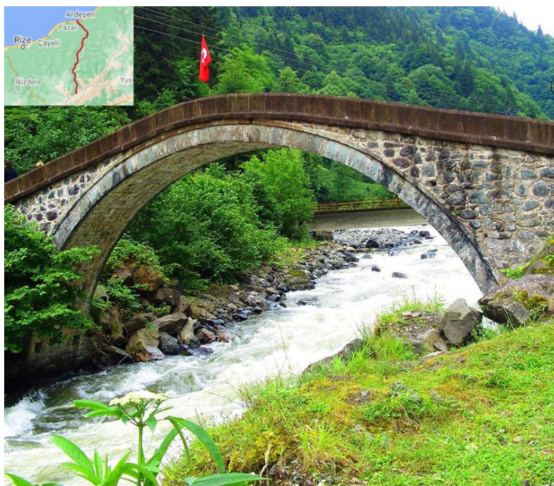
Figure 13. Firtina River and one of the historical arch bridges (Anonymous, 2022h).
