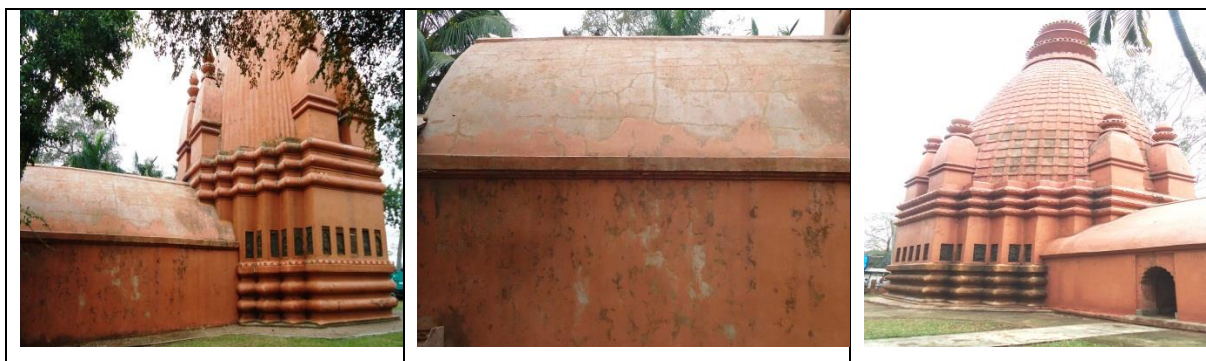
Fig. 2. After scientific treatment and preservation of North-East monuments (Images are self-explanatory results after preservation of lime plaster monuments).
